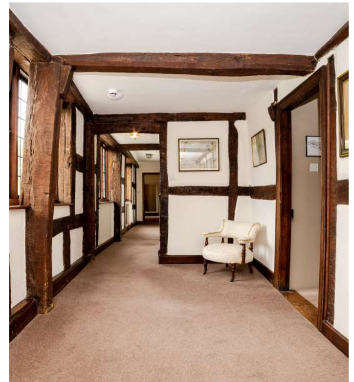
Broadfield Court, Herefordshire (2022) © Owen Hicks Architecture Image credit: Jay Watson Photography
